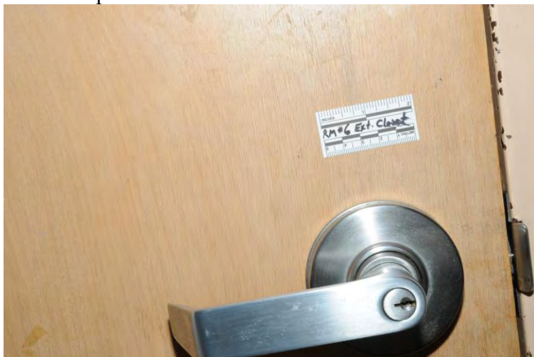
135 Example classroom closet door lock – exterior
