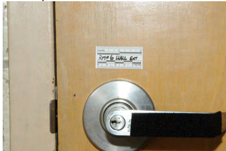
138 Example classroom door lock – exterior
