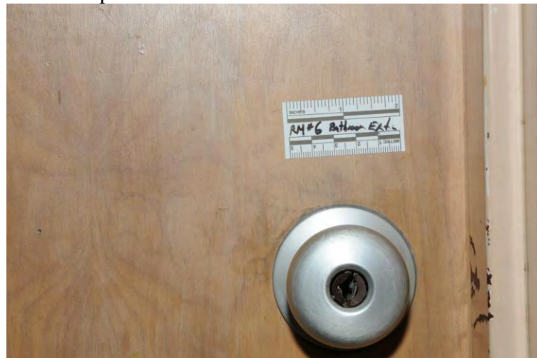
132 Example classroom restroom door lock - exterior
