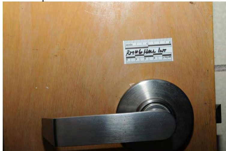
137 Example classroom door lock – interior
