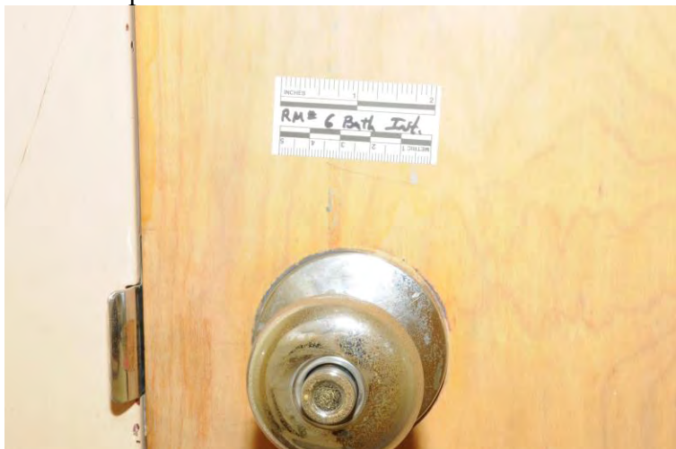
131 Example classroom restroom door lock - interior
