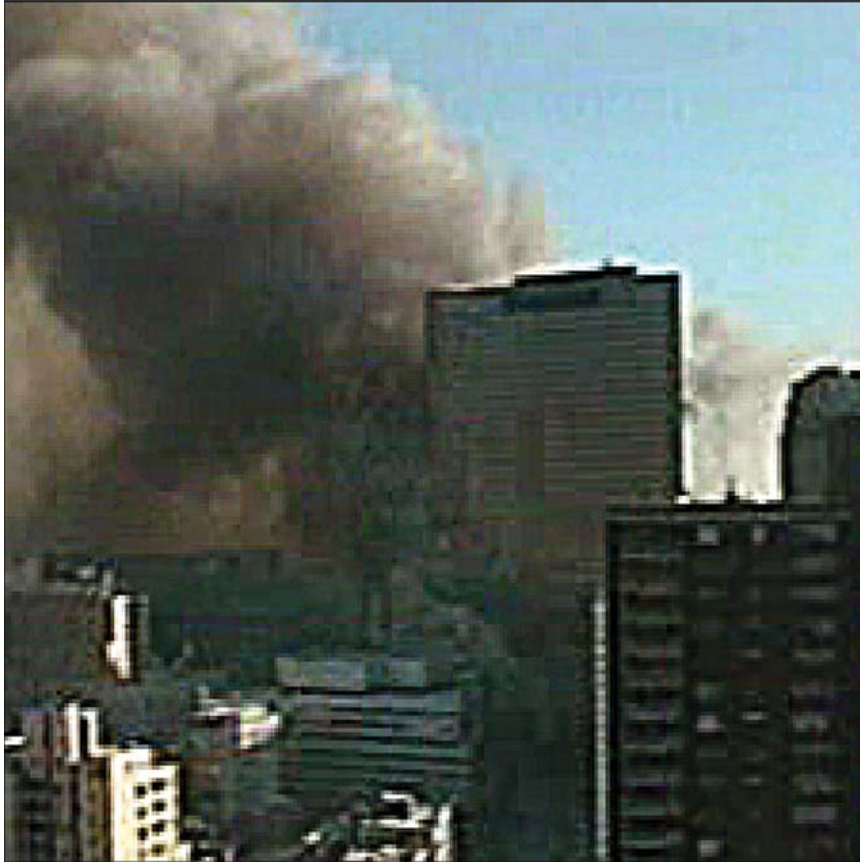
Figure 5-21 East mechanical penthouse collapsed. (From video.)
