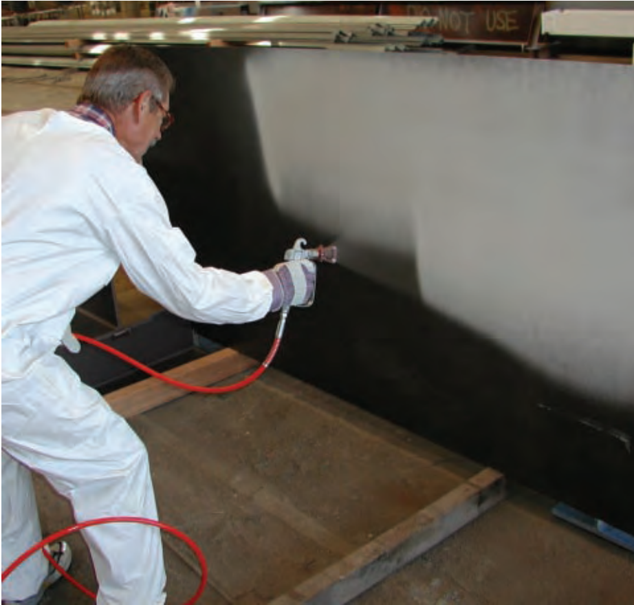
4: Applying the coating E-212-F to aluminium
