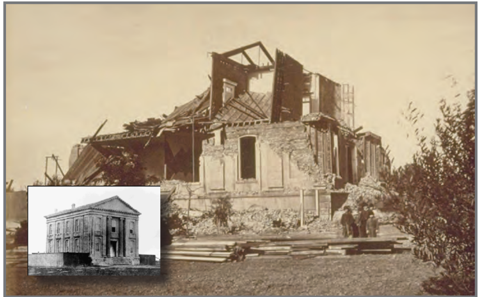
Strong shaking during the 1868 Hayward Fault earthquake caused the second story of the Alameda County Courthouse in San Leandro to collapse and severely damaged the building (photo courtesy of the Bancroft Library, University of California). The inset photo shows the building before the quake (photo courtesy of San Leandro Public Library). The 1868 quake devastated several East Bay towns and caused widespread damage in the San Francisco Bay region.
