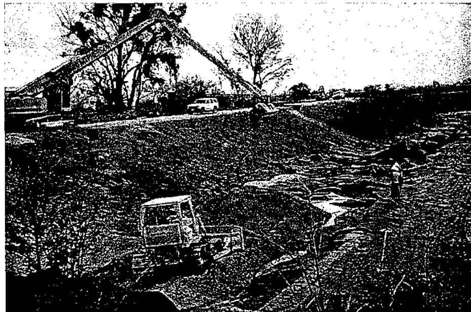
Emergency Flood Fight Repairs to a Distressed Levee along the San Joaquin River During the 1997 Floods.
