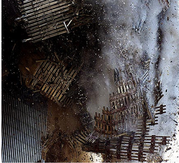
Figure 24. Prefabricated columns of the exterior wall falling to the ground completely detached from the floor structure.
