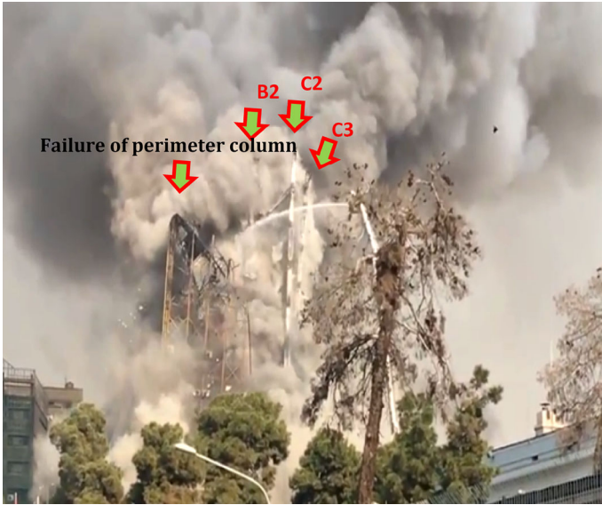
Figure 30. Appearance of the columns B2, C2, C3 and the collapse of the perimeter columns.
