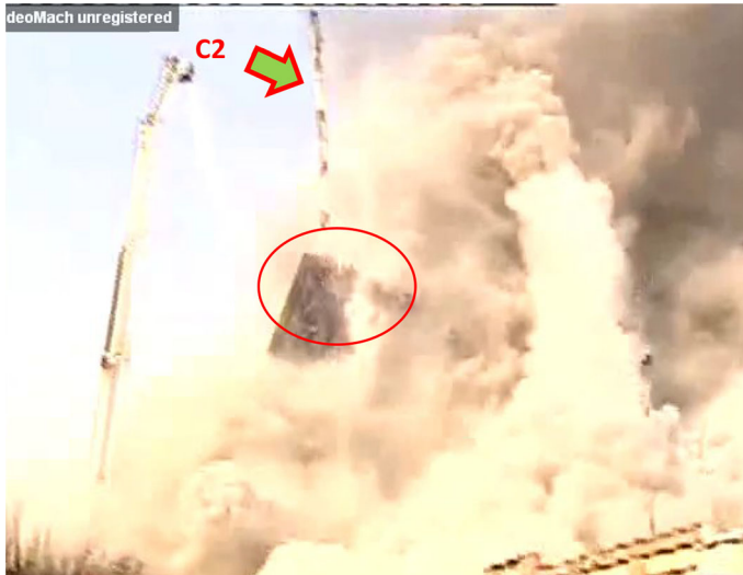
Figure 32. Overturning of column C2.
