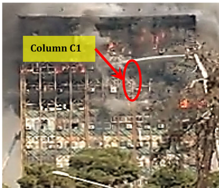
(a) After the appearance of the second fire bubble
