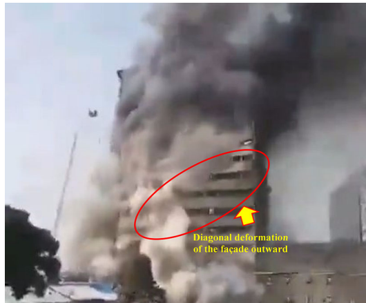
Figure 25. Non-uniform out-of-plane deformation a few moments before final collapse.
