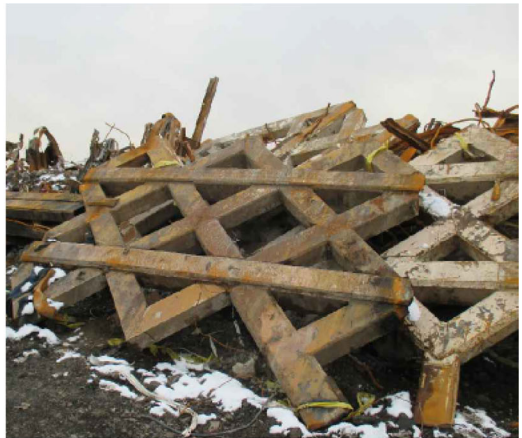
(b) Facade members built up with heavy steel sections
