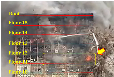
(a) Collapse of the floor 12 (first bubble)
