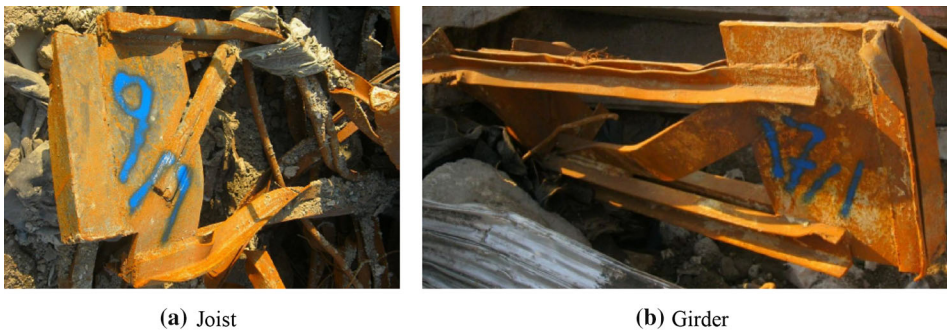
Figure 9. Floor joists and girders.
