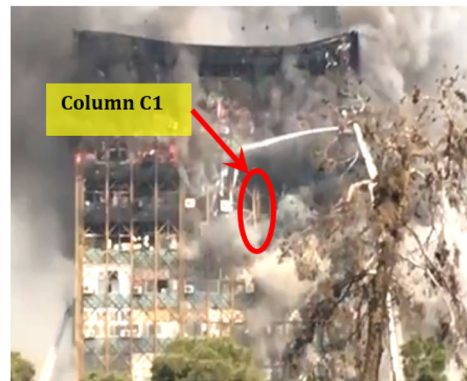
(b) Decoupling of the two parts of column C1
