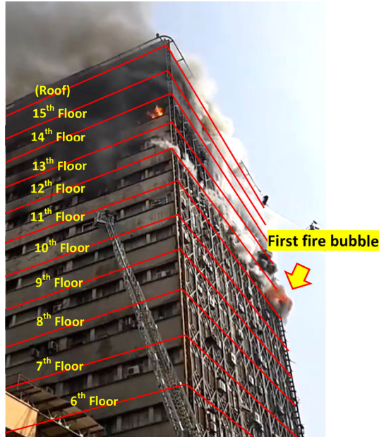
Figure 15. Appearance of the first fire bubble in the 11th storey.
