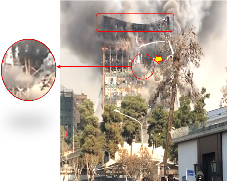
Figure 29. Progressive collapse of the south view of the building.
