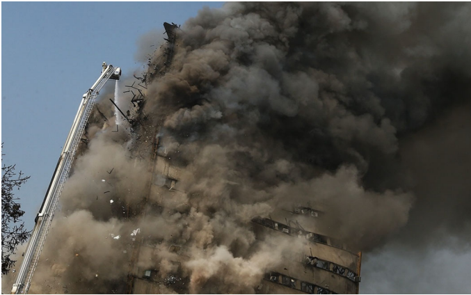
Figure 26. Final collapse of the entire building.
