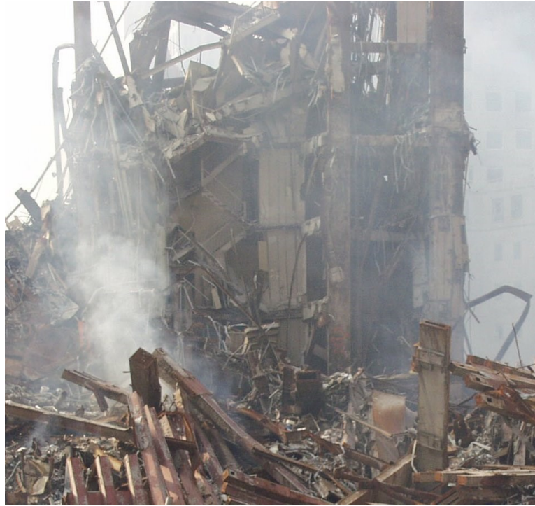
Figure 45: Close-up of the survivor's stairwell during debris removal. The stairs can be seen along the inner wall of the elevator shaft / core area.
