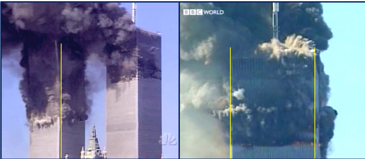
Figure 30: South Tower starts to lean (left) and North Tower starts to lean (right)
