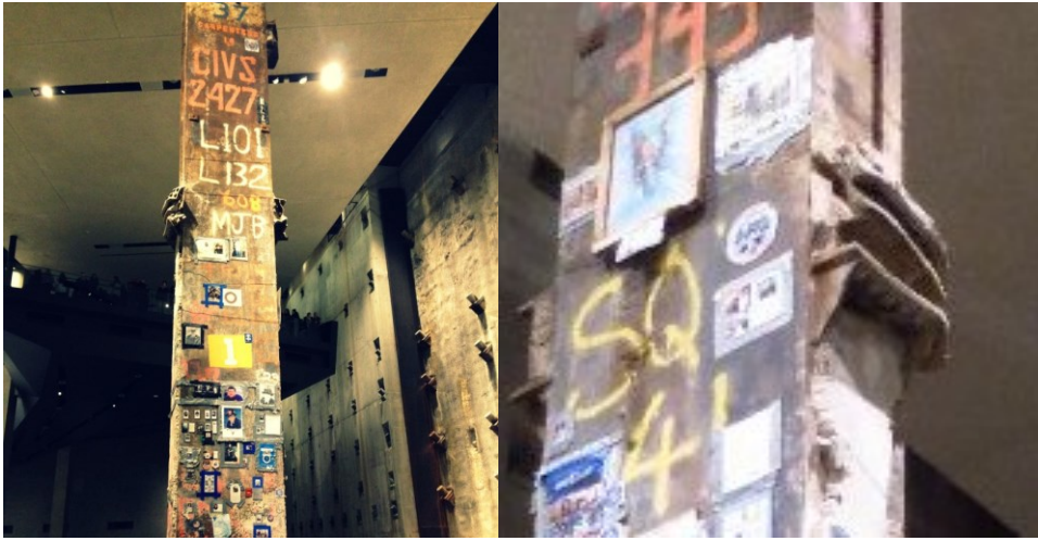
Figure 47: The "Last Column" was from the lowest level in the basement and shows the downward bend in a seat caused by falling debris that is characteristic of "Zone 3" damage.
