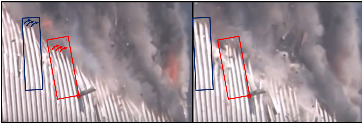
Figure 34: Rebound of the perimeter column sections after probable connecting bolt failure.
