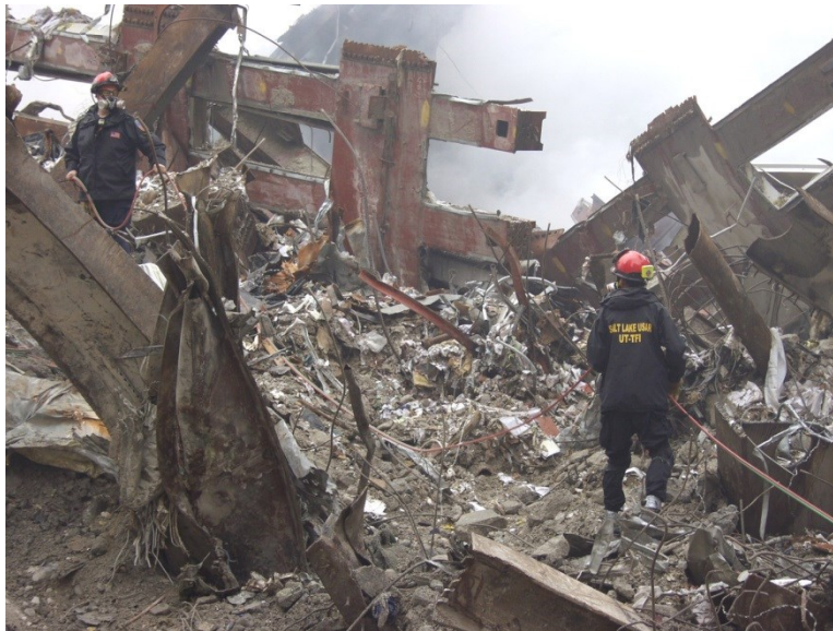
Figure 41: New York, NY, September 20, 2001 -- Rescue workers from the Utah Task Force-1 Urban Search and Rescue team prepare debris to be cleared at the World Trade Center crash site. Photo by Mike Rieger/ FEMA News Photo
