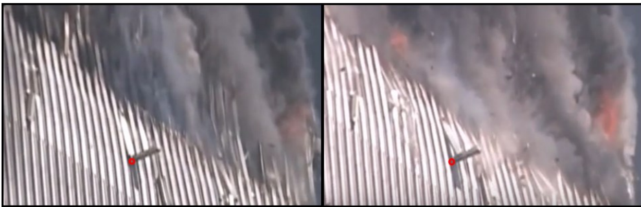
Figure 33: Push-in of the exterior perimeter columns by the hinged upper block as it begins pivoting/rotating.
