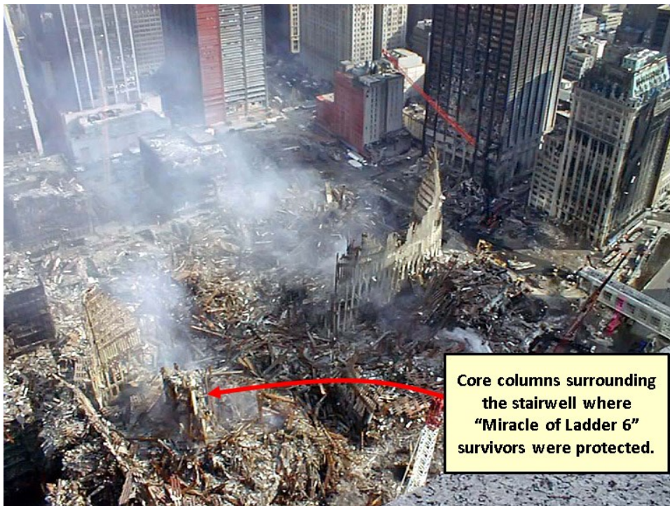
Figure 44: Post demolition view of "Zone 3" with the North Tower (left) and South Tower (right) with the core columns protecting the survivors in the 4 th floor stairwell identified by the red arrow.
