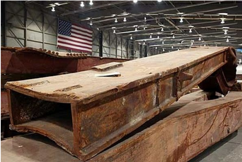
Figure 36: Core column with double concave bends in plates on opposite sides (Photo by Lane Johnson)
