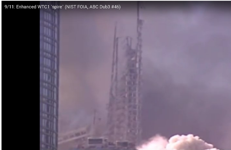
Figure 6: The "Ghost Spire" consisting of remaining core columns in the immediate aftermath of the destruction of the North Tower
