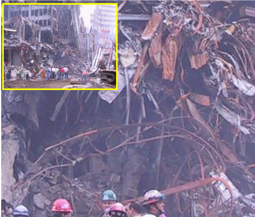
Figure 39: The only identifiable floor truss observed in photographs of the WTC debris field
