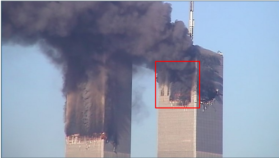
Figure 56: Relatively clear image of the eviscerated perimeter columns and missing floors in the area perpendicular to the core columns.
