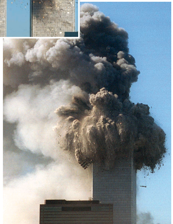
Figure 1. Flames and debris exploded from the World Trade Center south tower immediately after the airplane's impact. The black smoke indicates a fuel-rich fire (Getty Images).
