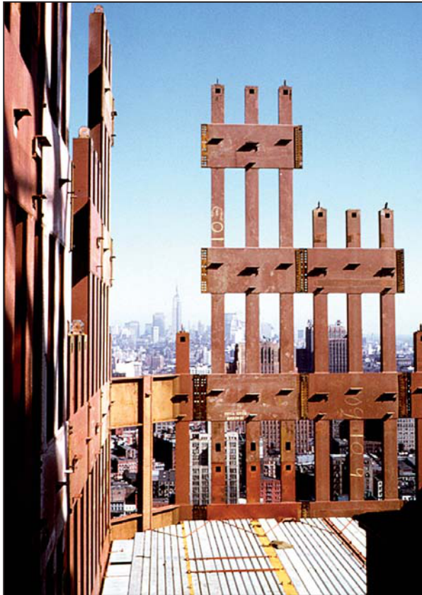
Figure 2-7 Erection of prefabricated components, forming exterior wall and floor deck units.
