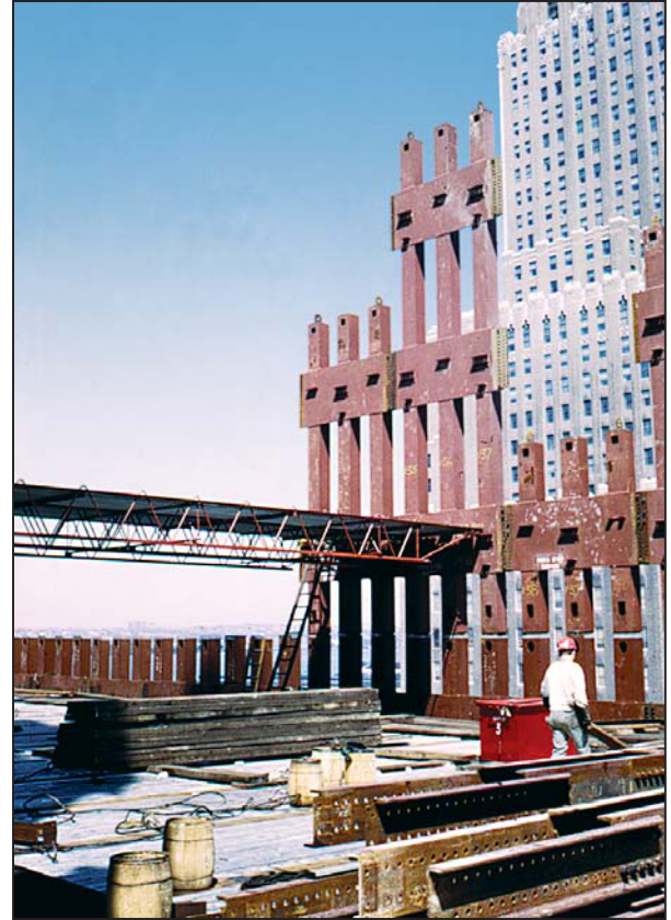
Figure 2-8 Erection of floor framing during original construction.
