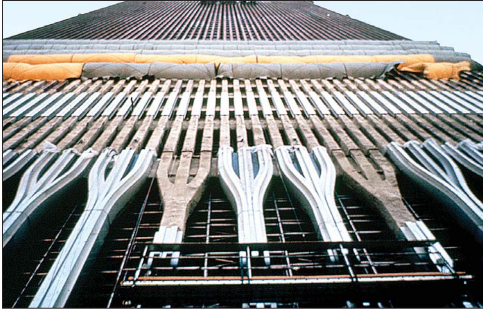
Figure 2-4 Base of exterior wall frame.
