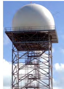
Figure 3.1-1: A Tower-Mounted Emitter
