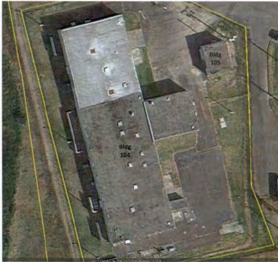
Enclosure 5. Present Condition of Building 104
