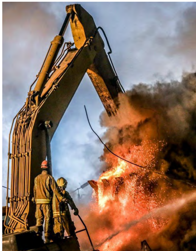
Figure 13: An excavator scooping up molten metal from the scene of the Plasco Building incident.
