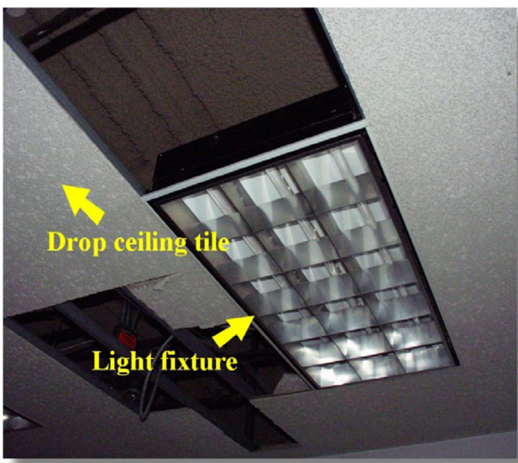
Figure 4. Typical drop ceiling used for above-ceiling samples
