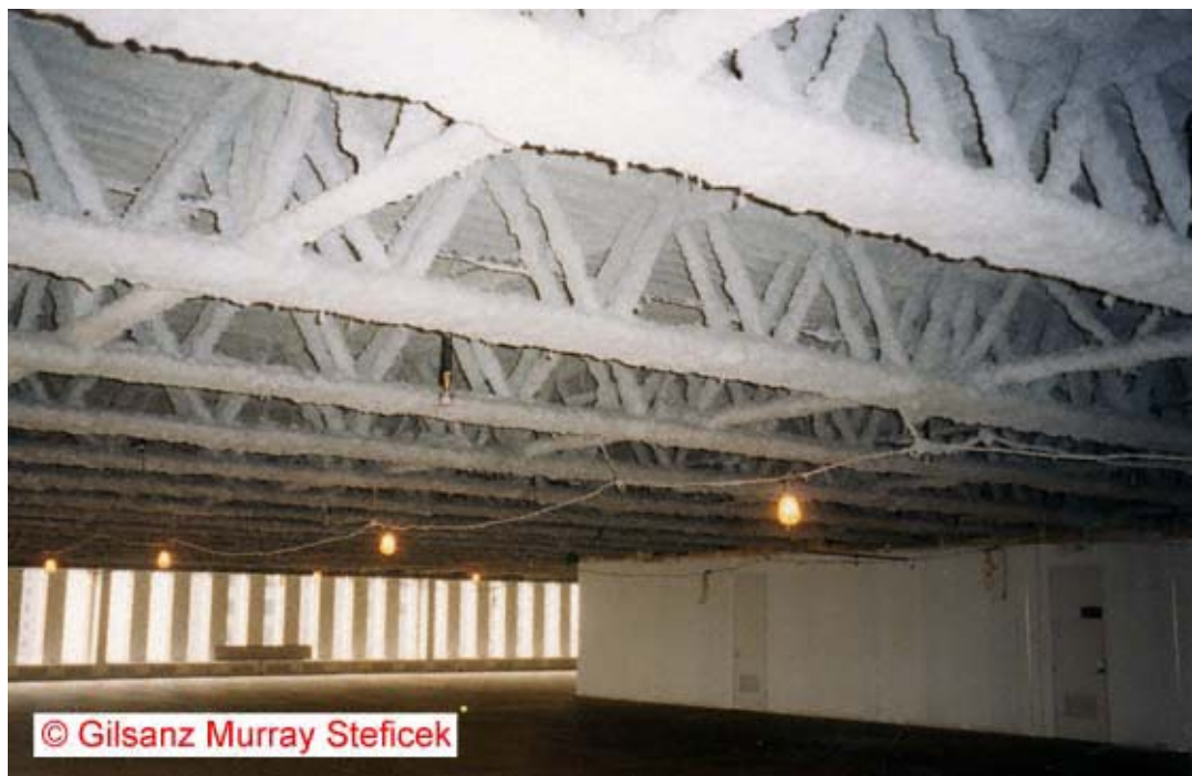
Figure 1–8. Photograph of insulated WTC trusses.
